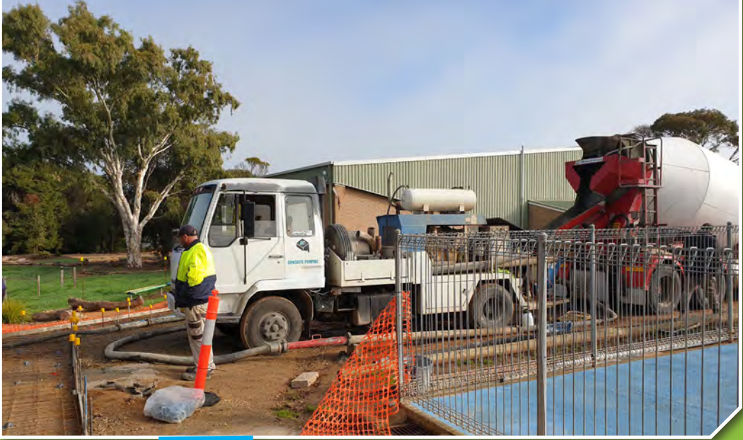
↓ The new Primary Oval footpath being laid.
